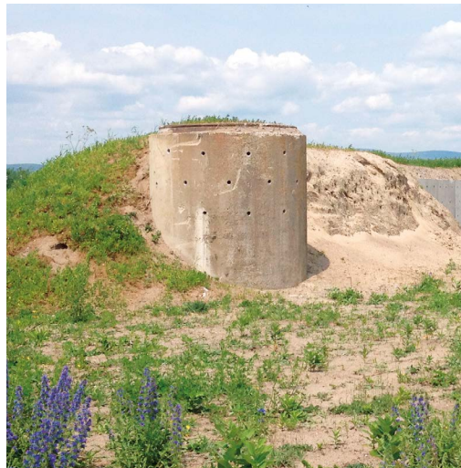
Vertical concrete pipes with premade holes.
